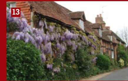
Apple Tree, Vine and April cottages on Church Lane looking east from Elmdene Cottage.
