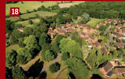
Bearley Green properties looking south-east from above the church.
