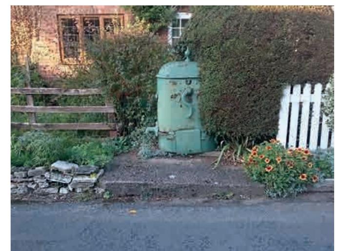
Dunstable Water Elevator in the village.
