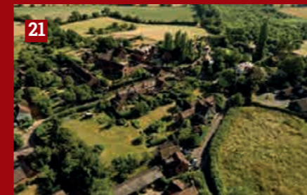
Church Lane heritage properties looking south from the church.
